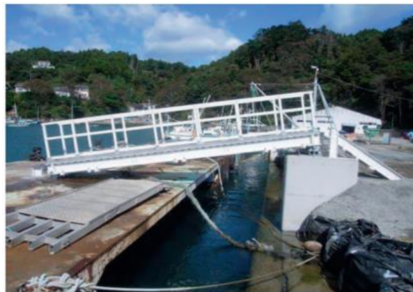
Figure 1.8: Glass Fibre Reinforced Plastic - Ultra High-Performance Fibre-Reinforced Concrete (GFRP-UHPFRC) pedestrian bridge in Miyagi, Japan [12]
