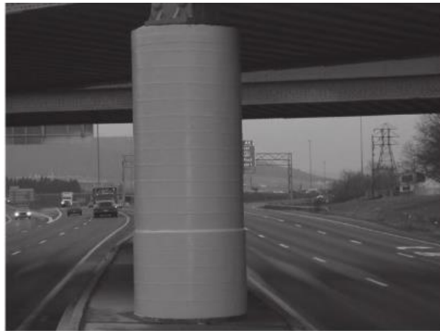
Figure 1.7: Repairing of a corroded concrete column by using fibre reinforced polymer [24]
