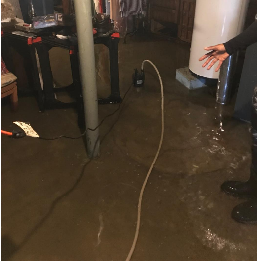
Figure 5.4: Flooded Basement in Detroit due to Combined Sewerage Overflow System
