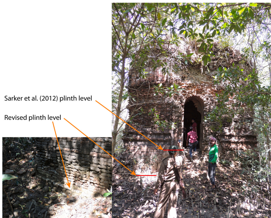
Fig. 7. Photo of the ~400 year old Shakher Temple in the Sundarbans with a closeup of our interpreted plinth level in the lower left.
