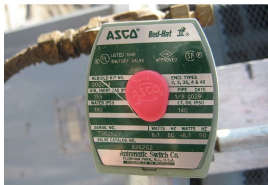
Figure 2. Nameplate for a typical automatic on/off valve for pump oilers
