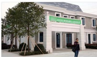
Figure 2-3. WinSun 3D Printed Mansion (~ 1100m<sup>2</sup>), in China (Stampler, 2015)
