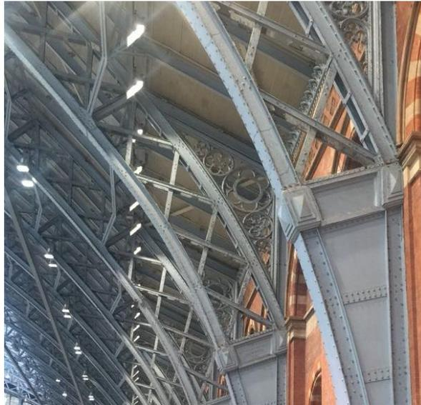
Figure 1-1. wrought iron frames in the roof of St Pancras station
