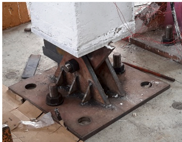
Fig. 10. Supports provided for the Connection's Column.
