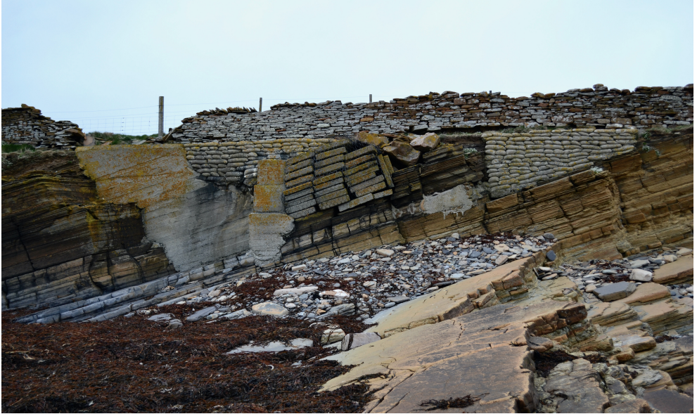
FIGURE 2 Varied concrete defences on Stromness' West Shore
