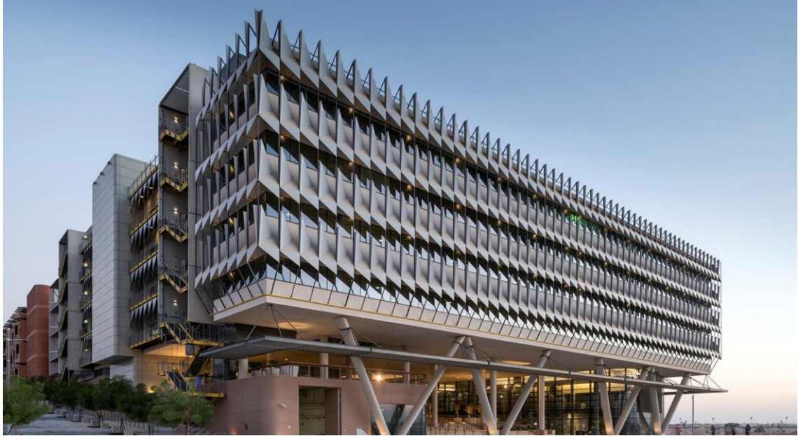
Figure 1.6: Siemens technology, Masdar City, UAE, designed with parametric optimisation of the façades for passive solar cooling and daylighting (AKDC, 2021).
