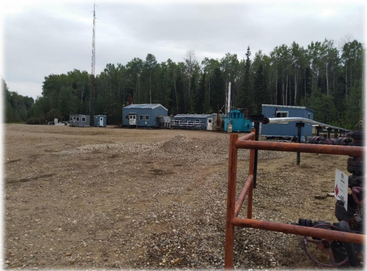
Figure 26 - An abandoned compressor station. Picture taken by Giuseppe Amatulli on September 26 th , 2019.
