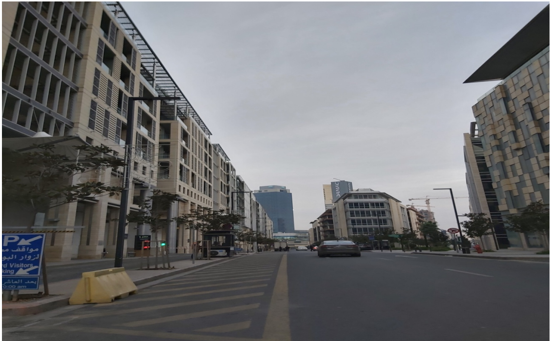
FIGURE 7.13 AL ABDALI AREA IN THE WEST OF AMMAN
