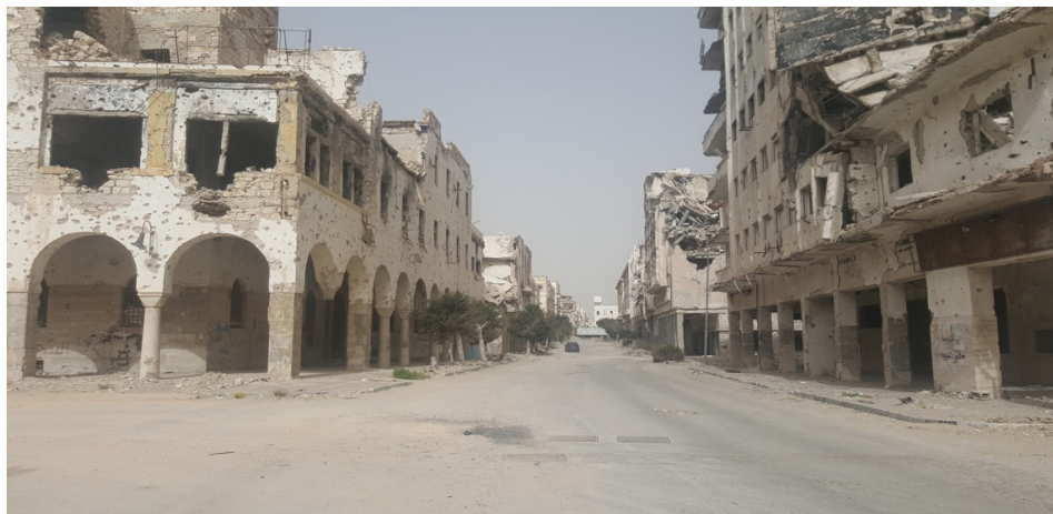
FIGURE 7.8 DESTRUCTION IN THE CITY OF BENGHAZI
