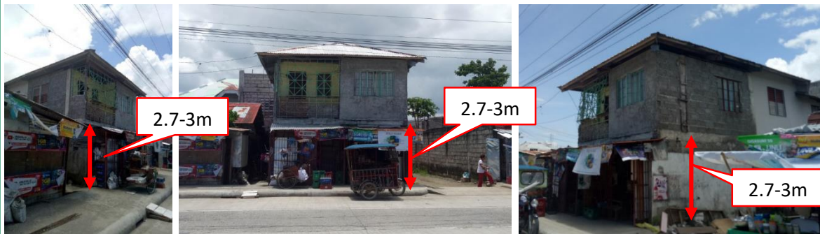
Figure 27: Actual photos of House E, with flood depth, located at Brgy. San Jose, Tacloban City, Leyte
