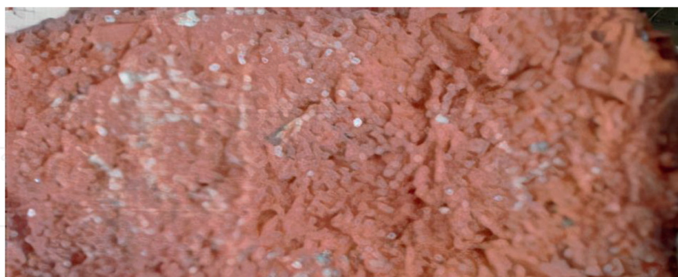
Figure 10. Brick after efflorescence test.
