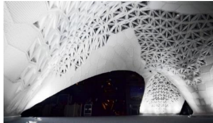
Fig. (10) VULCAN, architectural pavilion 3D printing Edg's printed for Beijing Design Week back in 2015 Park, Switzerland
