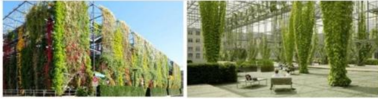
Fig. (8) Grid and wire-rope net systems, MFO Park, Switzerland
