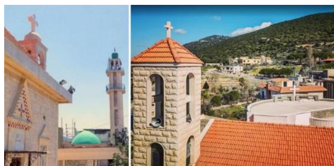
Fig. (18) picture showing Jarjough mosque and church
