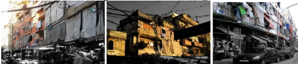
Fig.12: showing photographs of the exterior building conditions in Sabra
