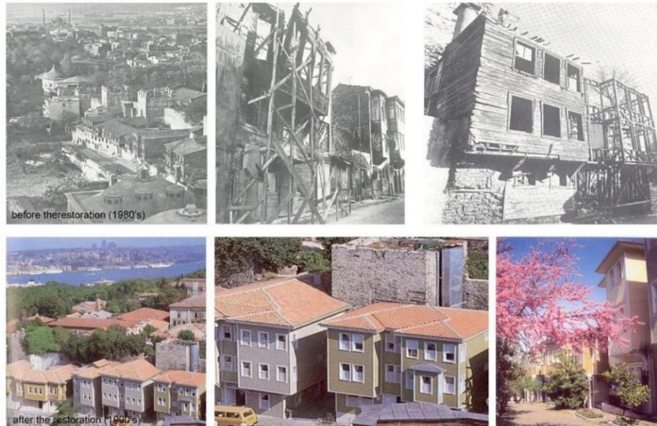
Fig.10: Sogukcesme Street before the restoration (1980's) and after the restoration (1990's) (Yenice. T & Altınoluk. Ü, 2019)
