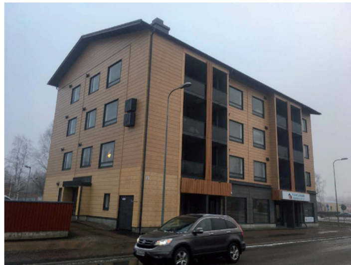
Figure 6. A four-story log apartment building ( Pinus sylvestris /Scotch pine), Pudasjärvi, Finland (Photo by Hüseyin Emre Ilgin).
