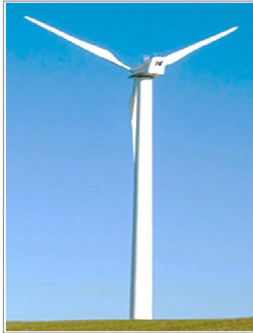
Figure 1. WindPact 1.5 MW Wind Turbine
