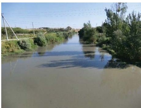
Fig. 2.1-2 A poorly maintained transport canal with turbid water in the Zeravshan River basin (August 2017)
