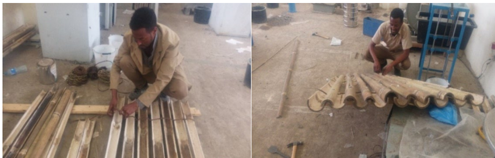
Fig. 6 - Fixing and constructing bamboo roof covering
