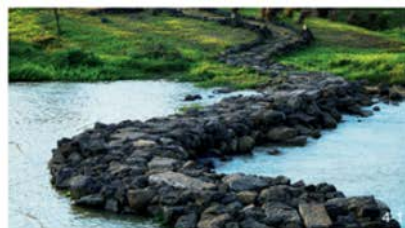
Figure 4-1. Volcanic stone snake bridge after completion.
