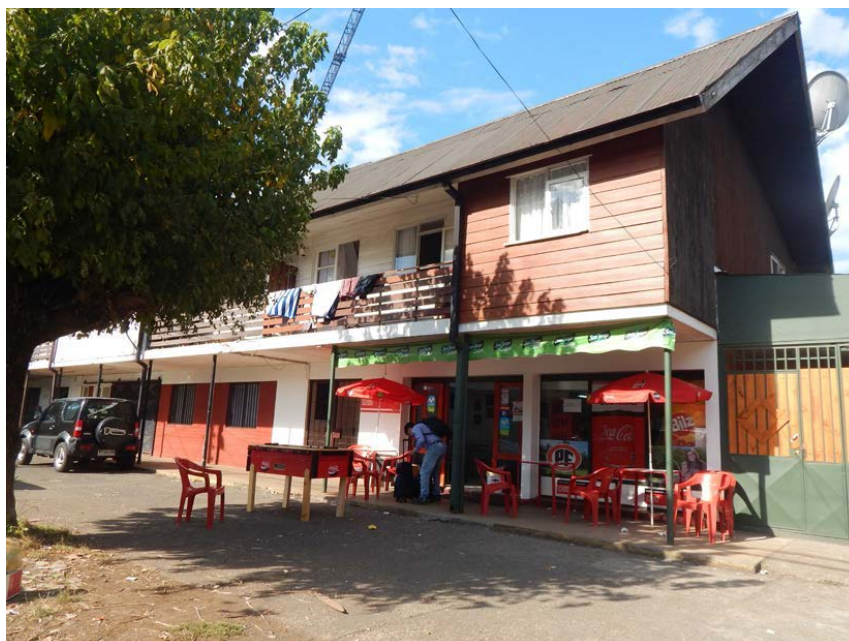
Figure 5. The house continues to be commercially renovated on the first floor.
