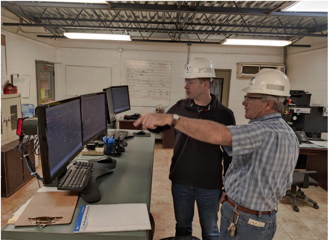
Figure 3. Maj. Mark S. Quint (left) and a member of the White Mesa staff examine the process control room at the uranium mill. During Operation Pay Dirt, Soldiers from the Aberdeen Proving Ground, Maryland-based Nuclear Disablement Team 1 trained at the White Mesa uranium mill in Utah and the Nichols Ranch in-situ recovery mine and plant north of Casper, Wyoming, April 4 - 8. U.S. Army photo by Col. John P. Kunstbeck
