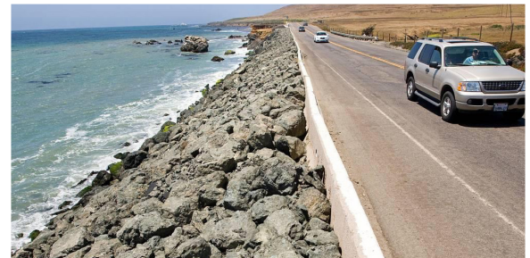
California Highway 1 before realignment, San Piedras. (Figure source: Caltrans).
