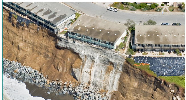
B. The same apartment buildings in Pacifica shown in Figure 5A in 2011 with failure of protection efforts prior to demolition (Figure source: Joel Avila, Hawkeye Photography).
