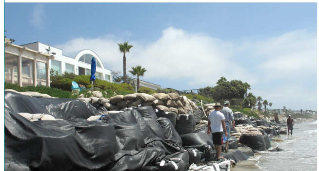
B. Broad Beach, Malibu (2008), with temporary sand bags, which didn't last a single winter and were replaced by a rock revetment (Figure source: Deepika Shrestha Ross).
