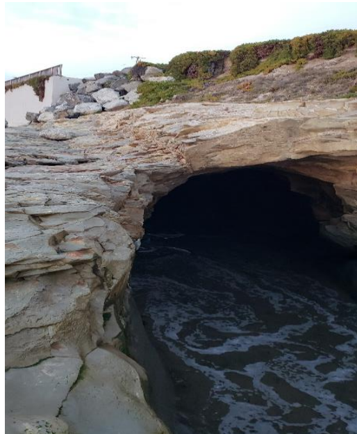
Figure 2-8 Cave Hazard near David Way in Zone 2.
