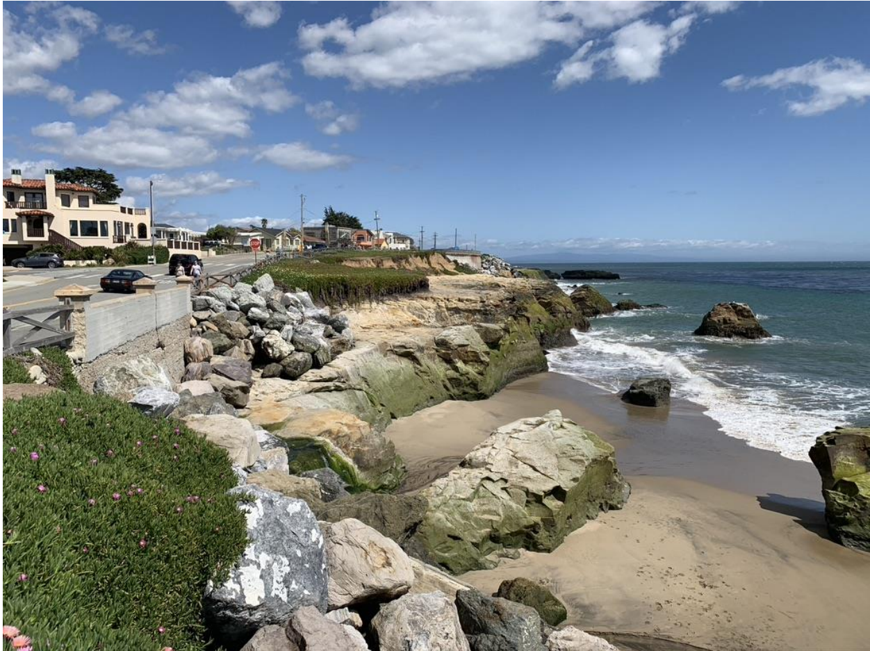
Figure 2-10 Seawalls along West Cliff Drive
