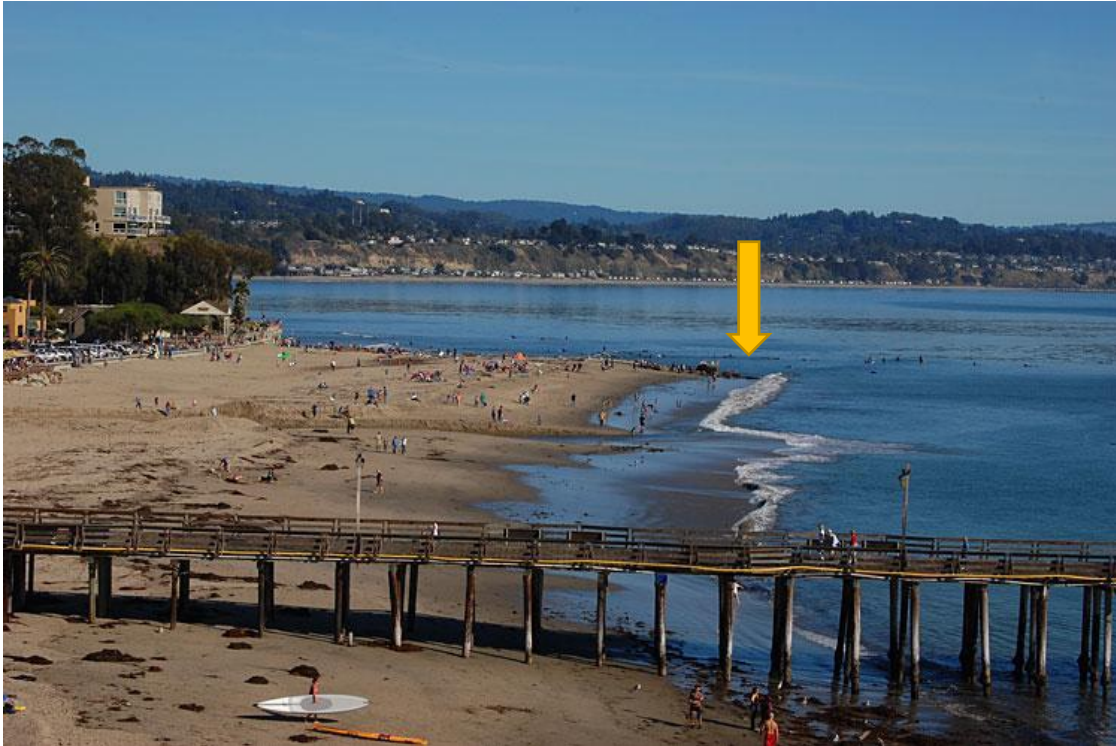
Figure 2-6. Capitola Village groin (in yellow) showing the widened recreational beach that also helps to reduce wave impacts.
