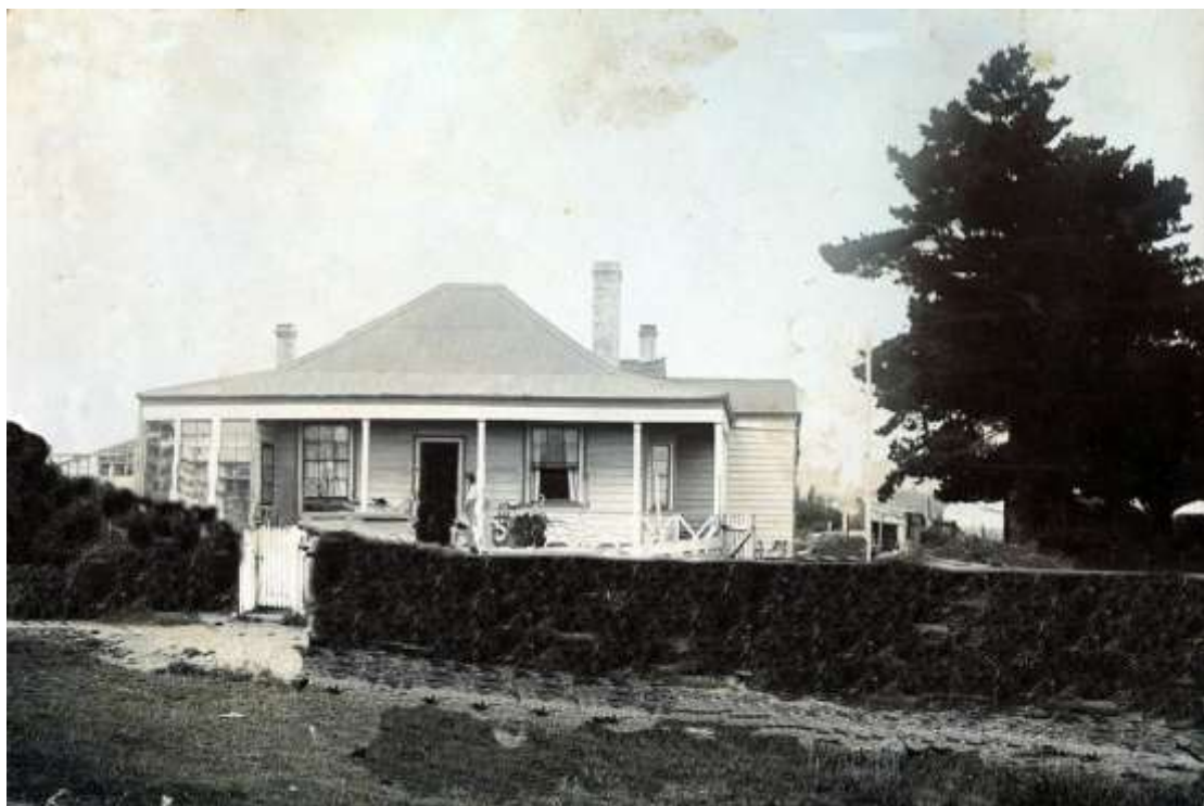
Figure 4. The Howell residence at Riverton, which was built in 1847. This photograph dates to 1907. Image reproduced courtesy of the Wallace Early Settlers Association.
