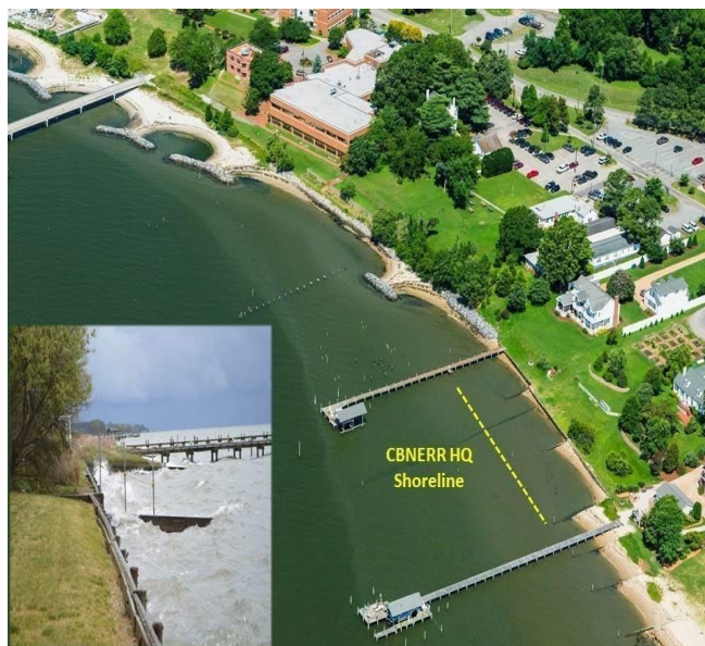
Figure 11.4. Aerial view of CBNERR-VA Headquarters highlighting location of failing shoreline protection infrastructure. Image sources: VIMS and W. Reay.
