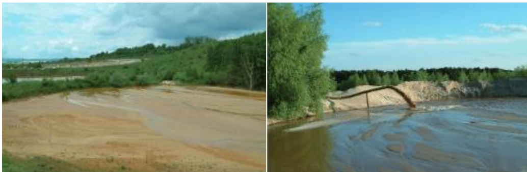
Figure 3-2: Typical disposal of AWS in ponds (Schmitz, Röhling & Dohrmann, 2011)
