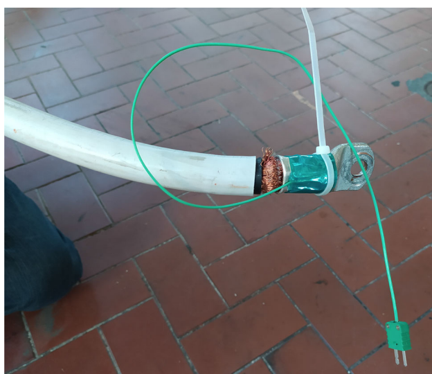
Fig. 15 View of the thermocouple place to measure the temperature rise of the lugs in the two tests
