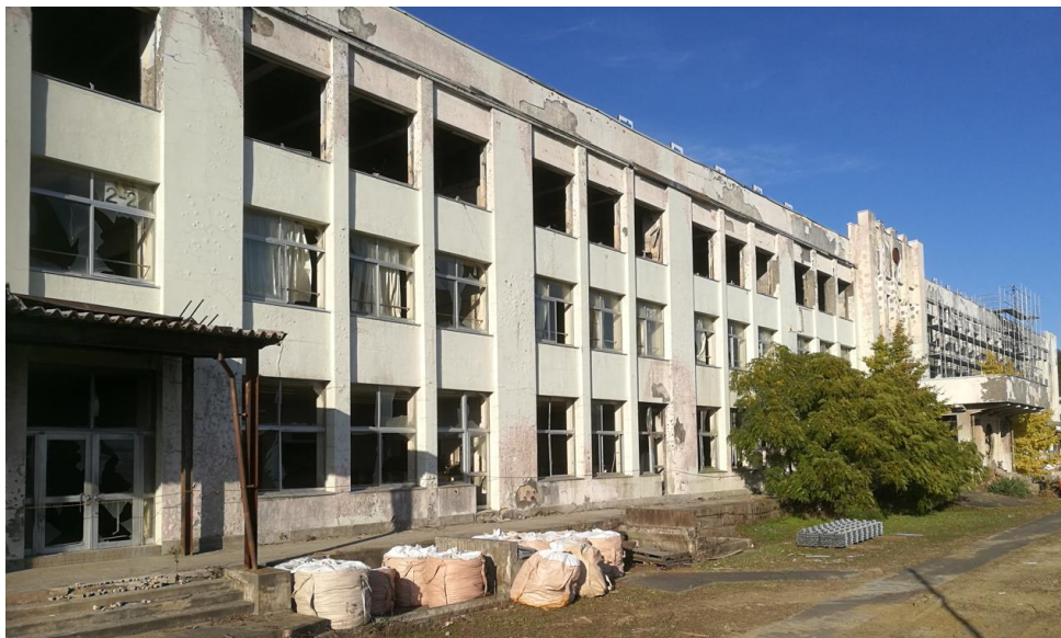
Fig. 12: Kodowaki Elementary school after being damaged by tsunami (November 2019)
