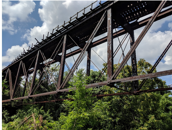
Failure/disruption during normal conditions due to e.g., extensive corrosion and deterioration
