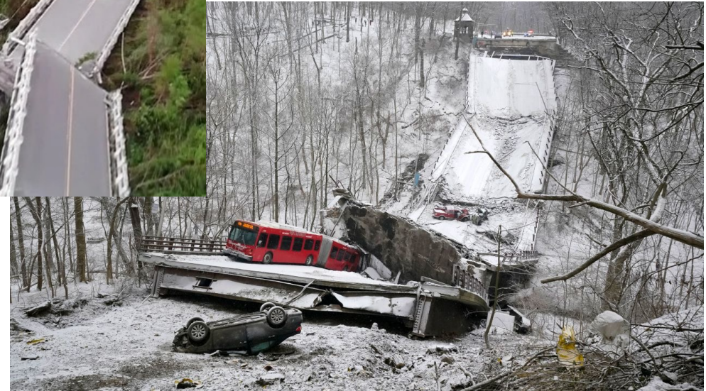
Bridge in PA collapsed due to lack of repair Replacement estimated at $25.3 mil https://www.cnn.com/2022/02/04/us/pennsylvania-bridge-repair/index.html
