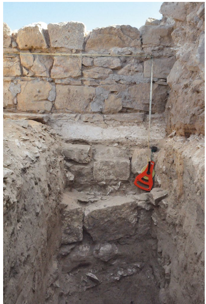
Fig. 31: Elusa (Halutza), peristyle building. Sondage 4, back wall of the northern portico. In the foreground stone foundations of an earlier mudbrick wall, looking NE
