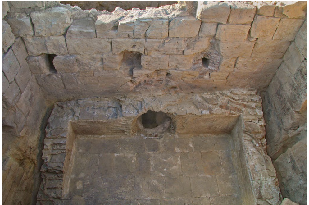
Fig. 39: Elusa (Haluzá), bath complex. Sondage 17, detail of the pool of the caldarium. The gap towards the praefurnium indicates a missing testudo
