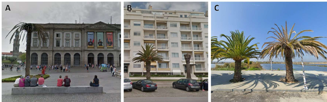
Figure 2. Damaged Phoenix canariensis palm trees in Porto, in front of the University headquarters (A) and in Avenida do Brasil (B), and in Aveiro in Rua da Pega in the vicinity of the University campus (C). Image C retrieved from Google maps.
