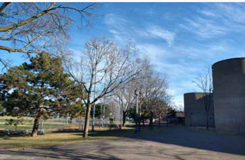
CURRENT BACK OF BUILDING AND SOFTBALL FIELD
