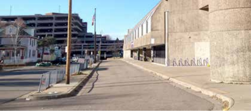
CURRENT SOUTH ENTRANCE
