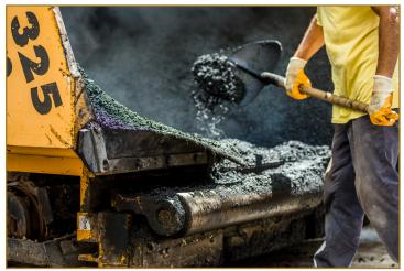
During paving works, HMA can stick tightly to instruments and tools.
