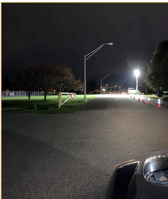
Roadway construction lighting systems.
