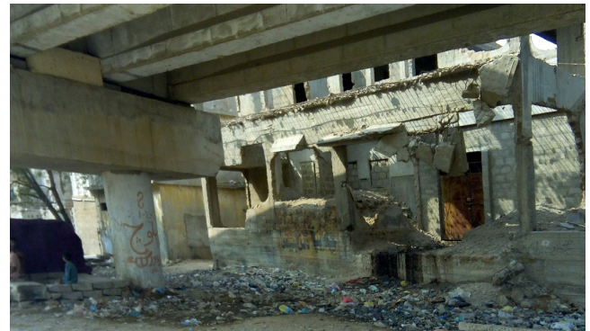
Picture of a partially demolished house in Salai Para
