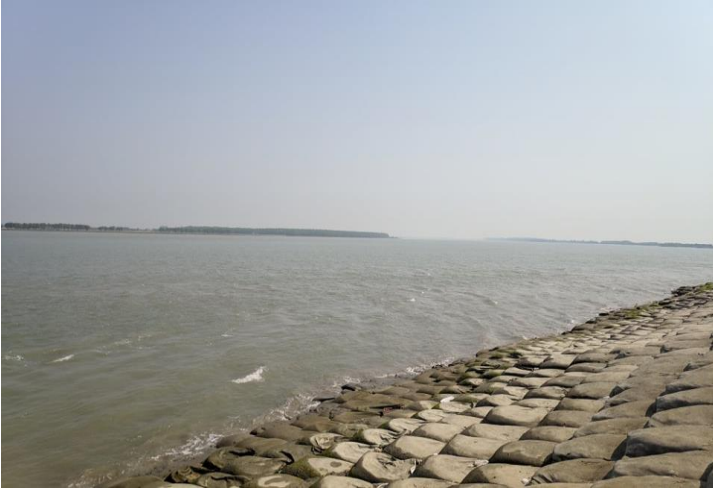
Erosion Protection Structure using GEO bag
