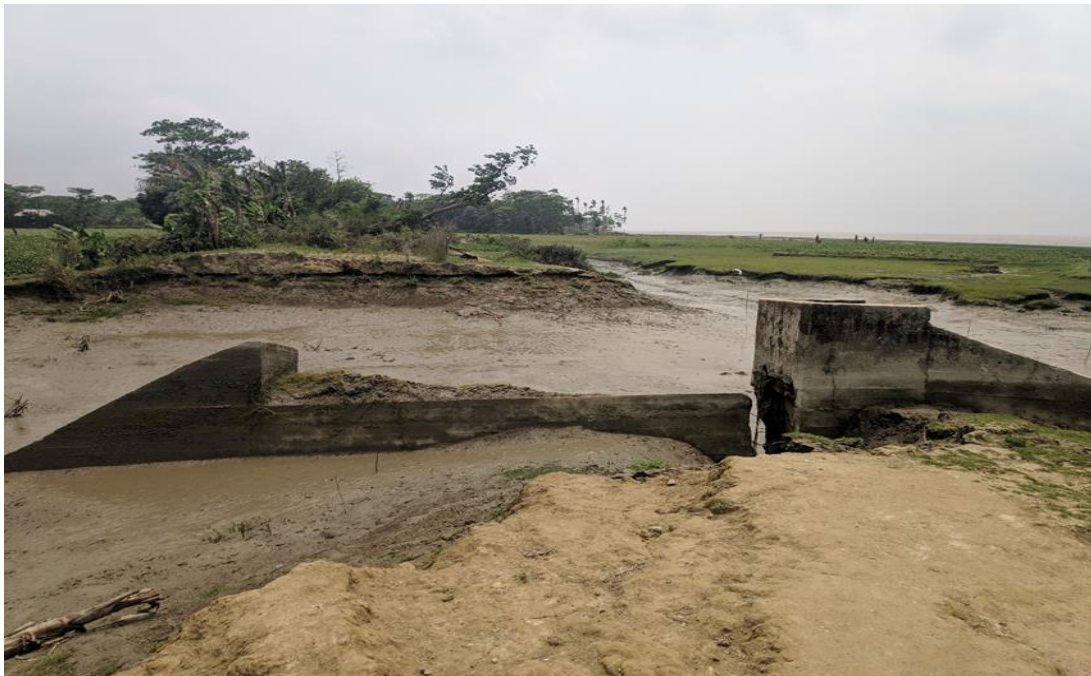
A vulnerable road in Raghunathpur village, Lakshmipur protected through geo bag.
