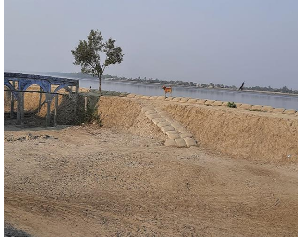
Erosion Protection Structure using GEO bag
