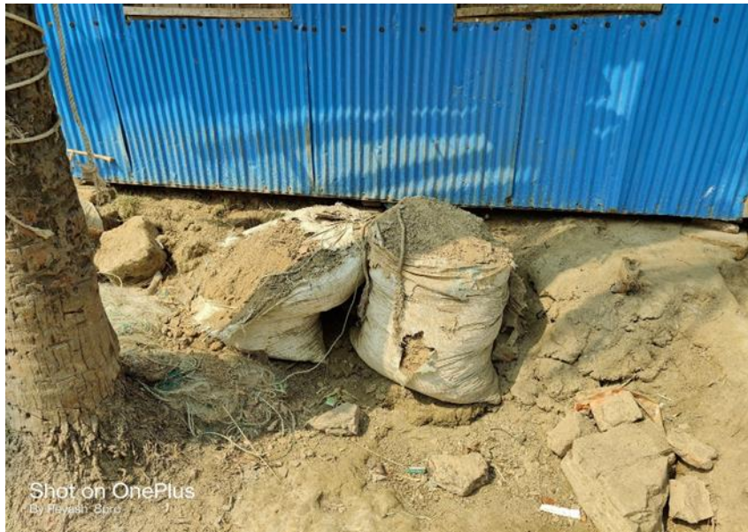
Raising plinth with geo bag are practicing as local adaptation in lakhshmipur
