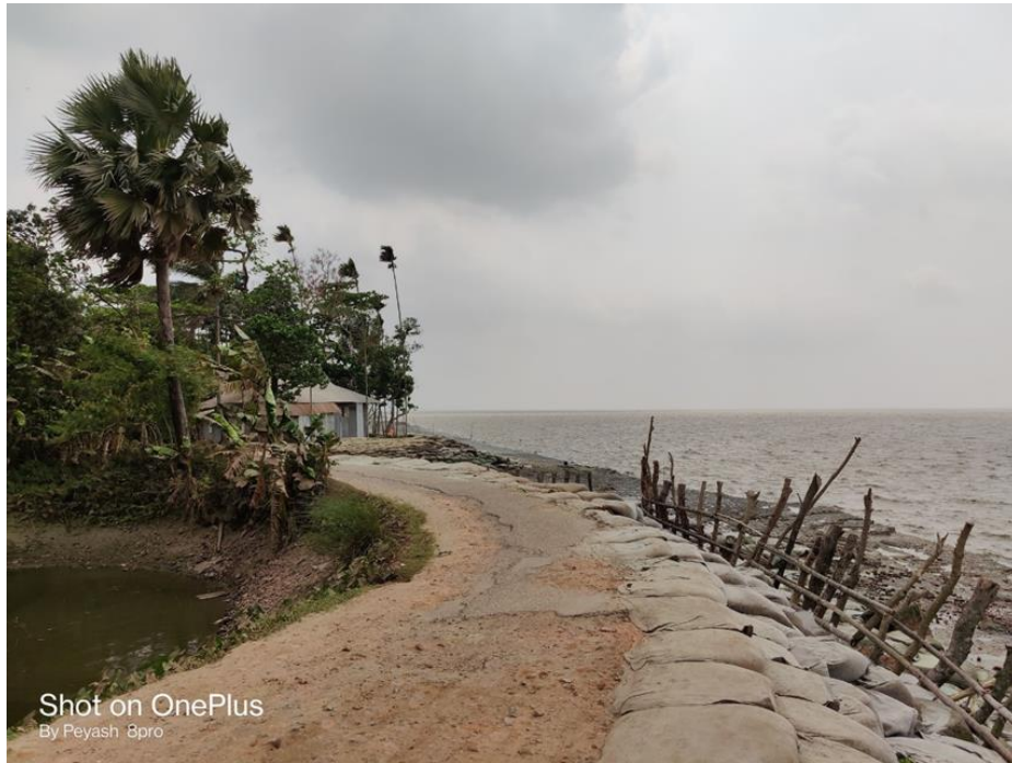
A vulnerable road in Raghunathpur village, Lakshmipur protected through geo bag.
