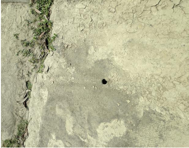
Number of rat holes are found in earthen embankment which reduces the durability of embankment. Rohita village, Barguna
