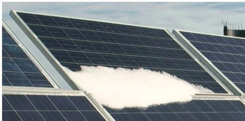
Figure 6.6 – TITAN PV module and the three substrings, each consisting of 20 solar cells. Image from the 27. March at 08:16, 08:39, and 09:21 with partial snow cover. Source: UiA PV System.
