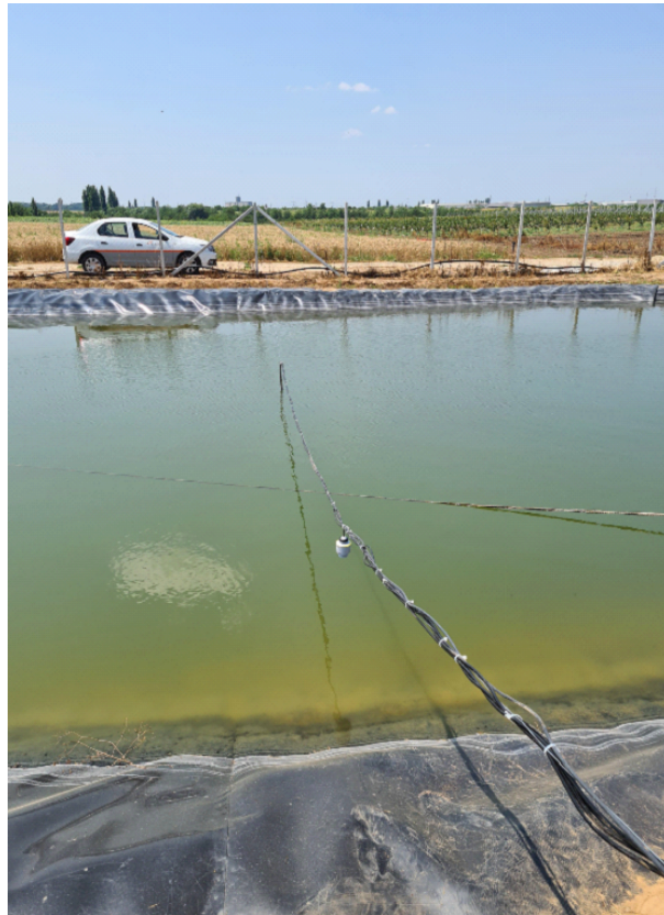
Fig. 2. Cables that connect to the sensor
