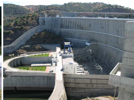
Alqueva Dam (Picture: Author)
