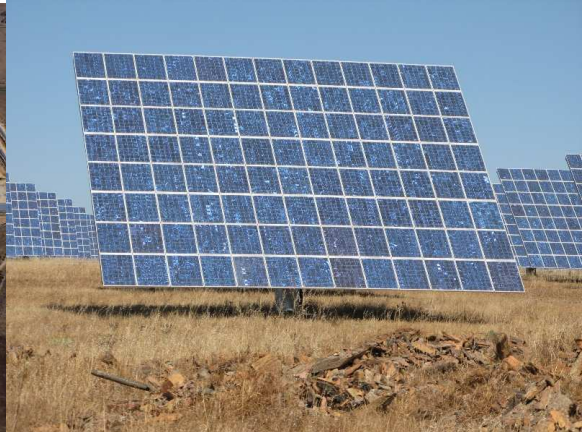
Photovoltaic System (Picture: Author)
