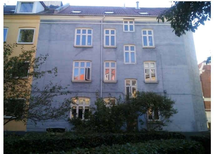
Fig. 15 View of the back facade, from the backyard
