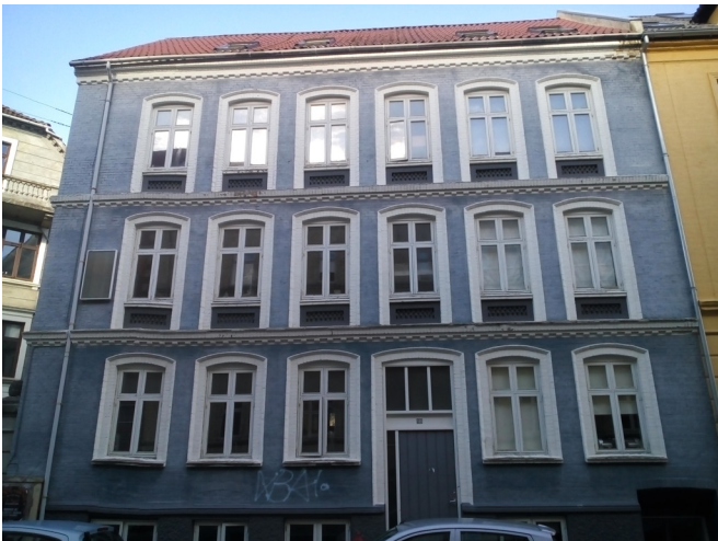
Fig. 14 View of the building front facade
