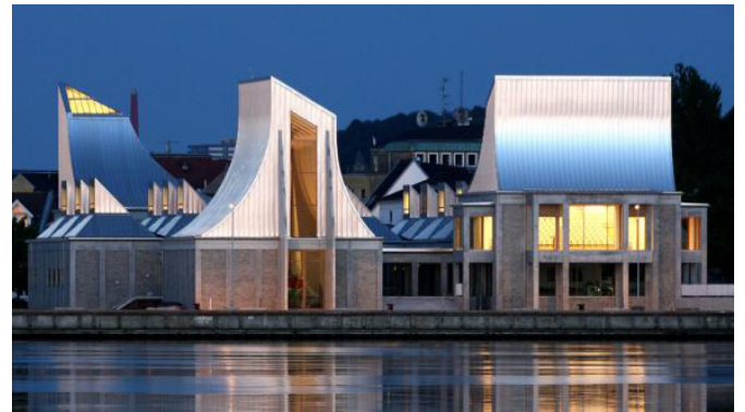
Fig. 7 View from the Fjord of The Utzon Centre, design by Jørn Utzon
