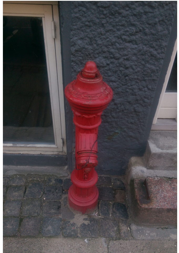
Fig. 18 Hydrant, near the front door, allowing easy access in case of emergency
