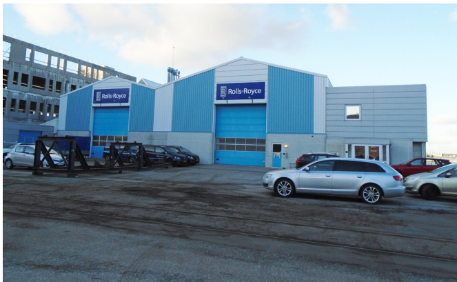
Fig. 100 Rolls Royce Service, on the West side of the site
