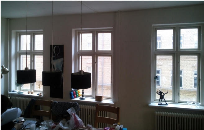
Fig. 23 Apartment windows are double layer and are in good state, if changed for new one will be to improve the acoustic.
