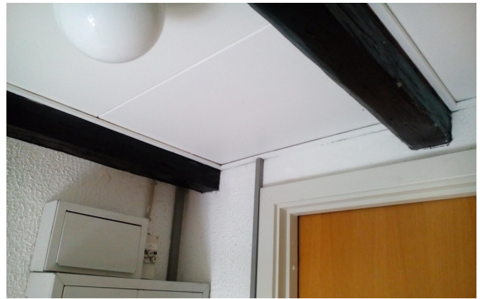
Fig. 29 The rafters are exposed and look like there is no damage in the building structure
