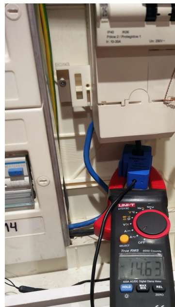
Figure 32. Calibration Process - Amperometric Clamp (14.63 A reading).
