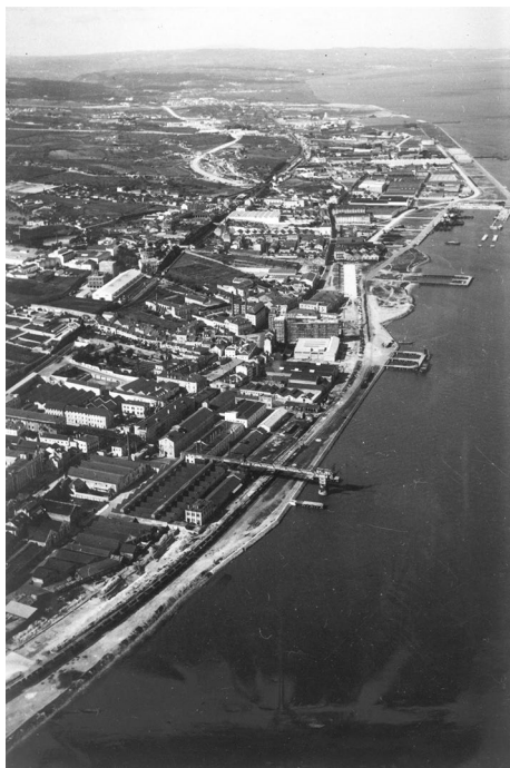
Fig. 3 Panoramic View of the industrial area in the eastern axis extending from Lisbon (1950). Source: Municipal Archive of Lisbon (PT/AMLSB/SPT/000195)
