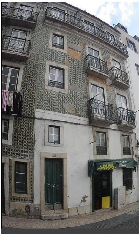
Building Front Side
