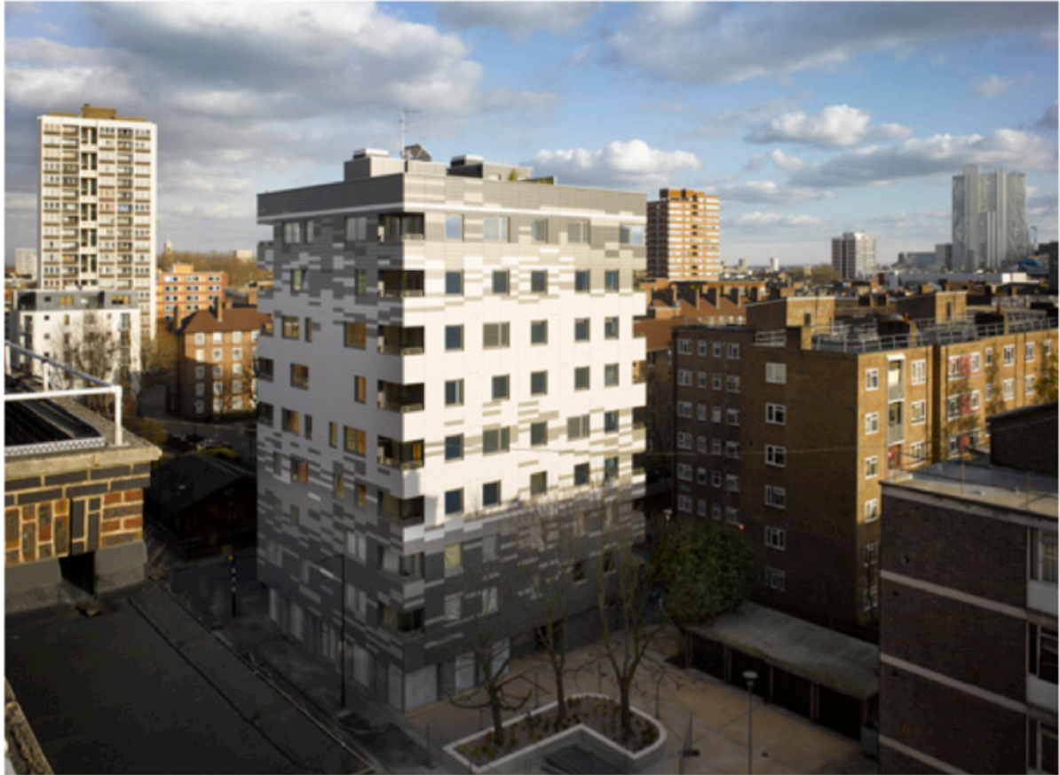
Fig.10 Stadhaus, looking west along Murray Grove, London, UK. [25]
