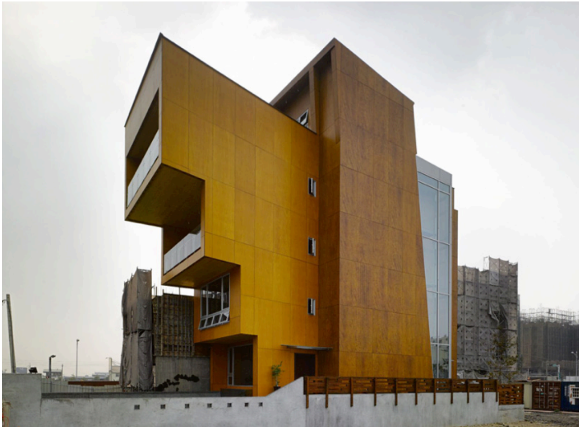
Fig.13 WoodTek headquarters, Taiwan, China [28]
