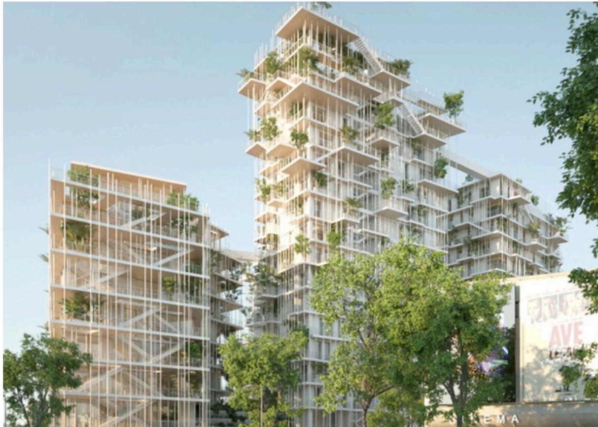
Fig.19 Bordeaux Tower – Bordeaux, France [34]
