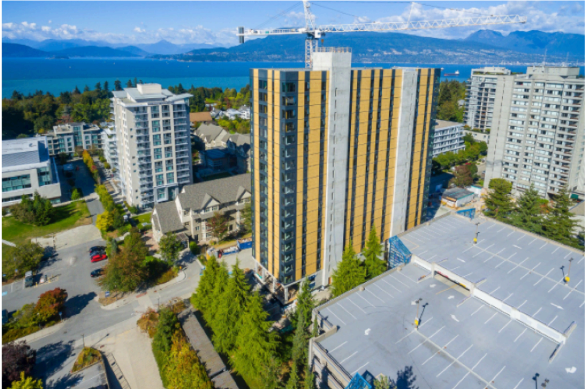
Fig.16 UBS BROCK COMMONS – Vancouver, Canada [31]
