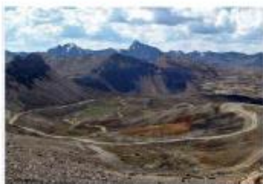
Tailings Storage Facility – Toromocho Project, Peru ($147 Mn):
