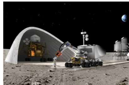
Fig. 76 - A Contour Crafting robot is shown here printing a road in front of a parabolic hangar structure housing a lunar lander. In the background, can be seen a plant intended for processing regolith that will be used in the construction process. Taken from nanowerk.com.
