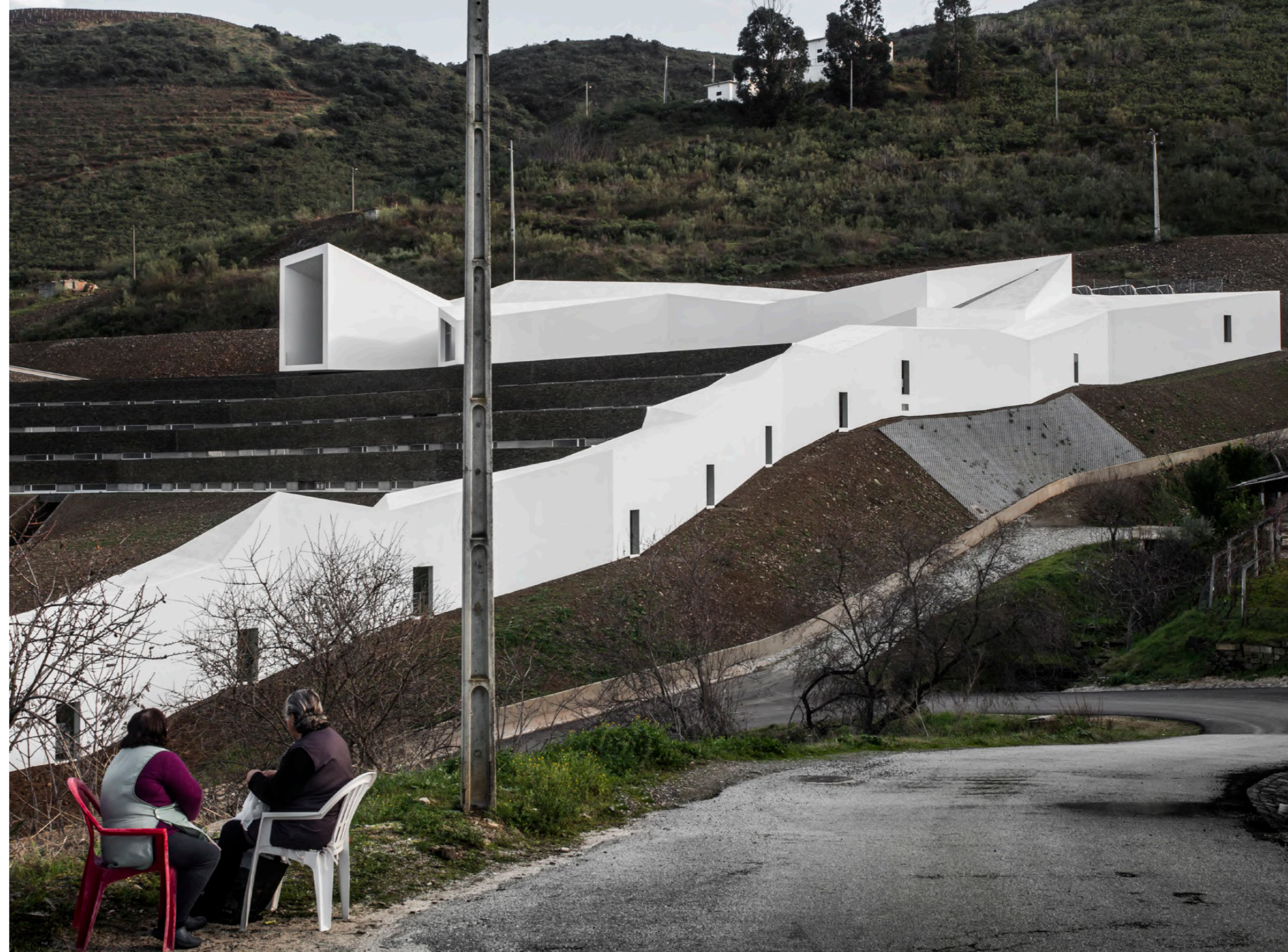
Fig XX - Part of the center for High Yield- Rowing Pocinho View (Fernando Guerra | FG+SG)
