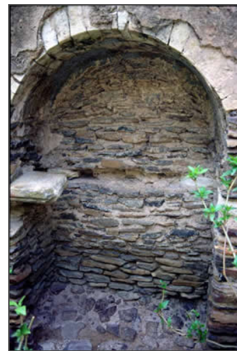
Dabsan ("house of the patriarch"), Niche (Photo: H. Pennec)
