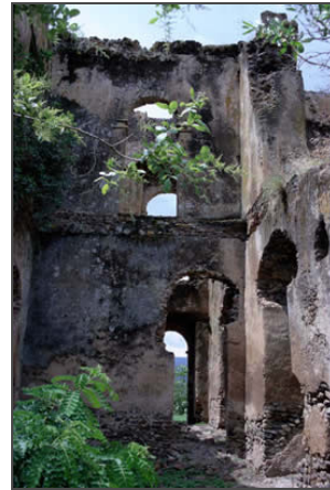
Dankaz royal palace, Interior (Photo: H. Penneç)
