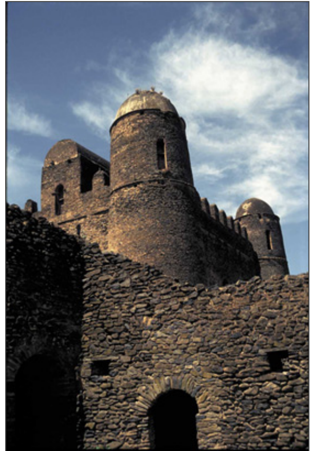
Gondar palace compound, Fasiladas' royal palace (Photo: H. Pennec)
