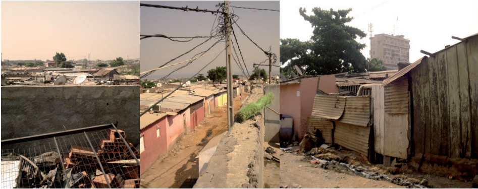
Figures 16, 17 and 18: Materials and construction quality of self-construction houses. Various aspects
