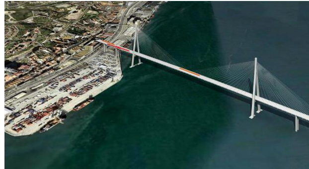
Figure 6 Photo montage of the North riverbank of TTT Source: LNEC (2008)
